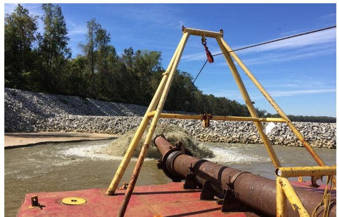
**Spillbarge discharges pumped sand behind newly constructed rock training dike at Jackson, AL**
